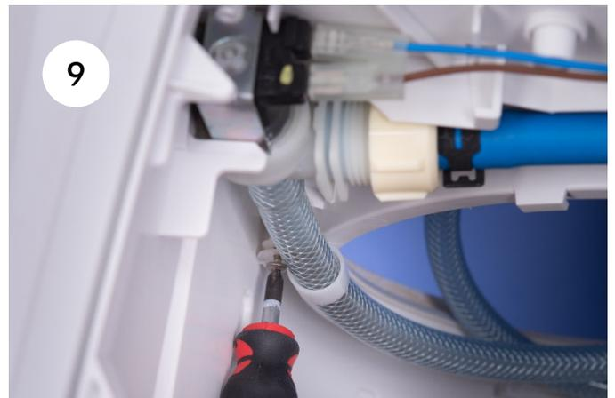
9. Unscrew the fresh water hose; it may be necessary to loosen the screws on the clamps.
